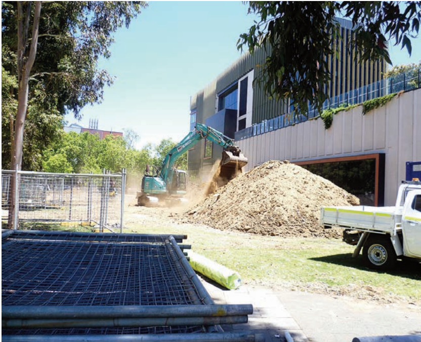
Construction works commence at Adelaide Botanic High School in January 2023.
